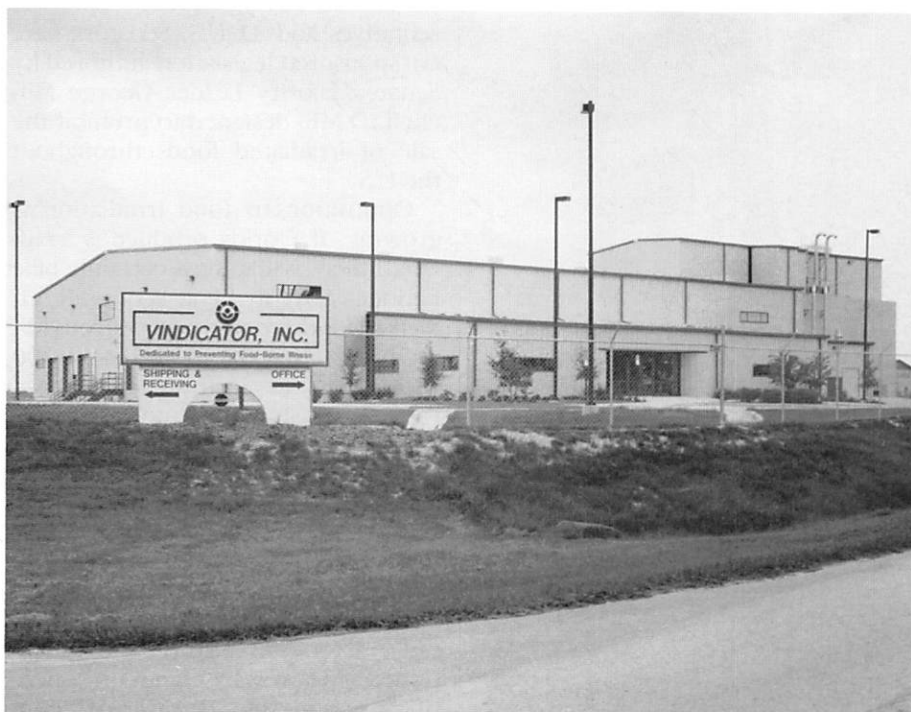
If ever opened, this food irradiation plant under construction in Mulberry, Florida, will begin irradiating Florida fruits and vegetables—if it can find farmers and growers willing to risk a national boycott of their products.
